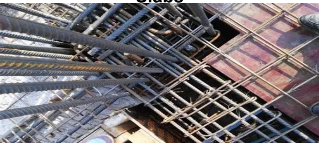
Prefabricated building frame column joint connection
